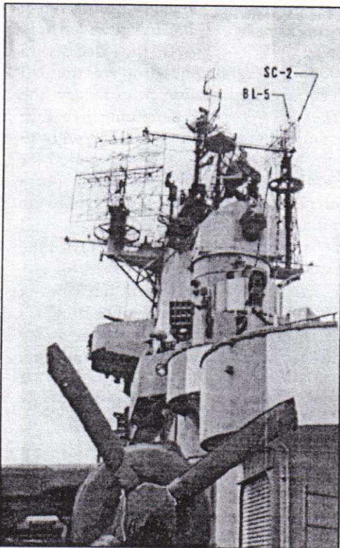
A Type D-1 Array: Two views of U.S.S. Yorktown in September 1944. The big SK radar has been moved aft to make room for an SM fighter-control set on the foremast.
