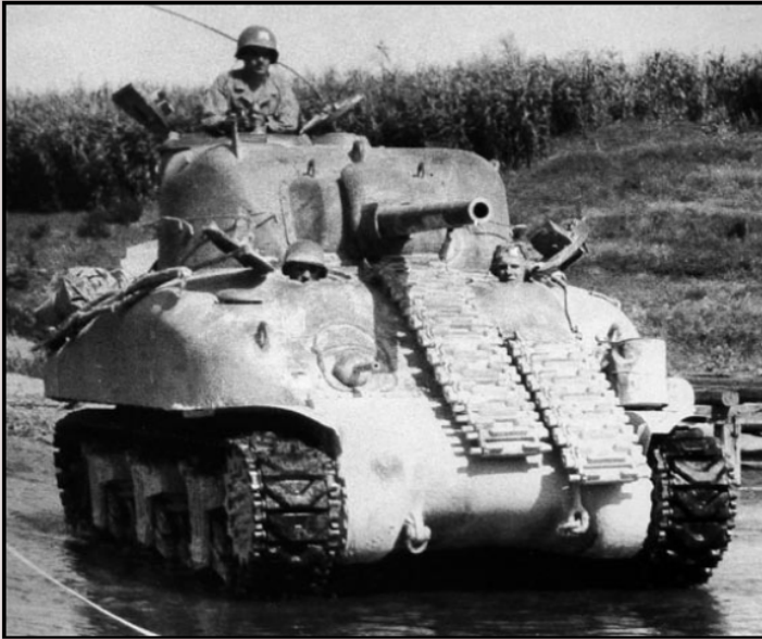
This M4A1 clearly show the rounded edges of the cast hull. The M4A1 was powered by the Continental nine-cylinder, gasoline radial engine.
