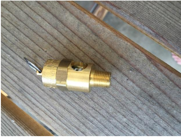
A 1/8" NPT 125PSI Safety Pressure Relief Valve
