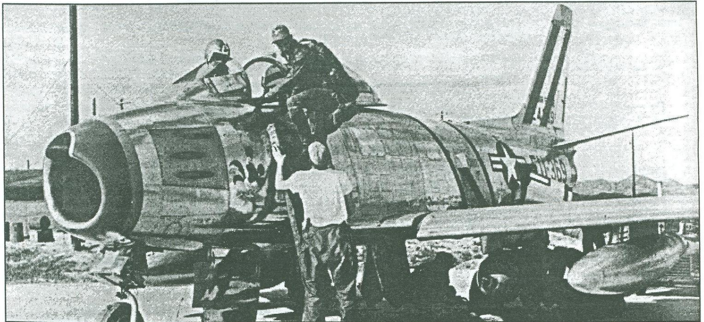
Pilot and ground crew prepare an F-86 for a fighter-bomber sortie. This photo depicts an "E" model with the slatted wing.
